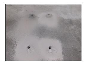
Clean holes with pressurized air or vacuum to remove any excess dust/debris
